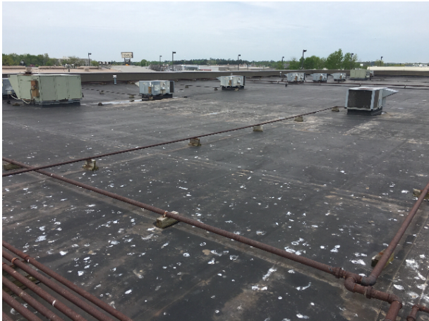
Section 6 Looking West towards Shopko
